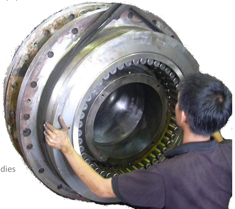
Installation of a spherical roller bearing
